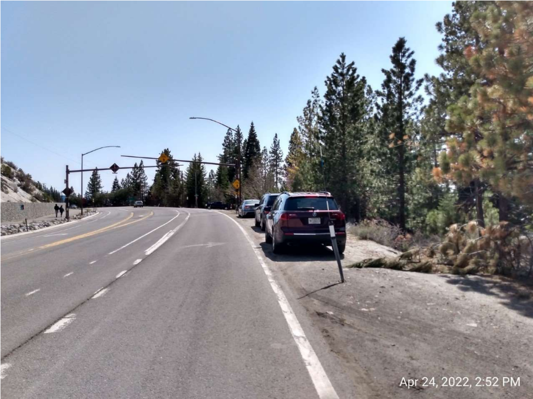
Parking in the No Parking zone beside the right turn lane onto Lakeshore.
