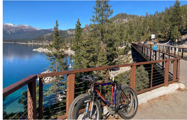
SR 28 LAKE TAHOE EAST SHORE TRAIL
